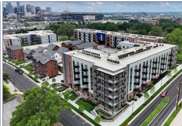
Park Point East, a new housing development featuring 203 apartments.
